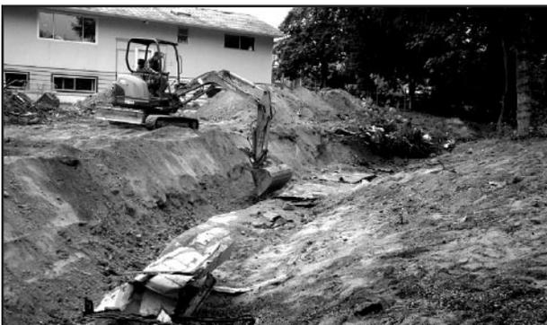
*The stream had been lined with metal frames and topped with sheet metal, which was then covered over with fill.*
